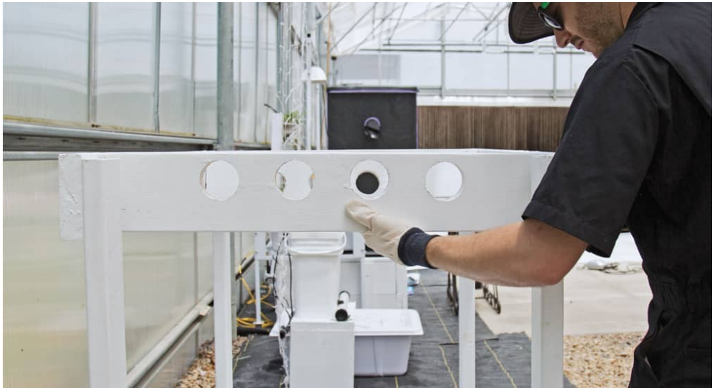
Crossbeam with drilled holes near the top
